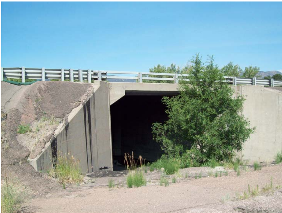
Photo 1 – View of Bridge Structure ID: H-17-AI.
